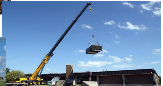
Building C HVAC project
