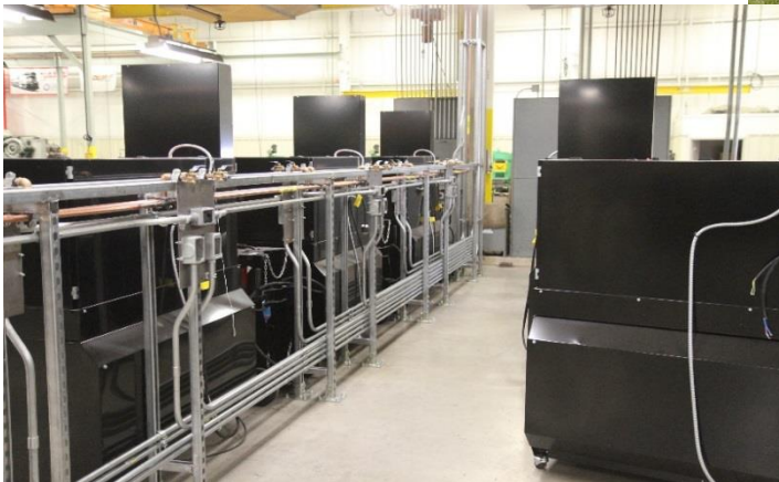
Welding Lab Expansion
