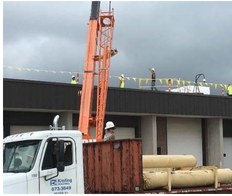
PHS – Building B Roof
