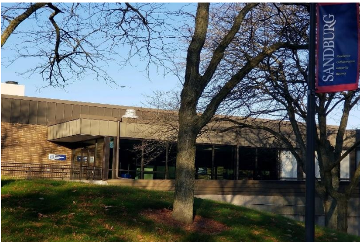
PHS Windows Bldg E
