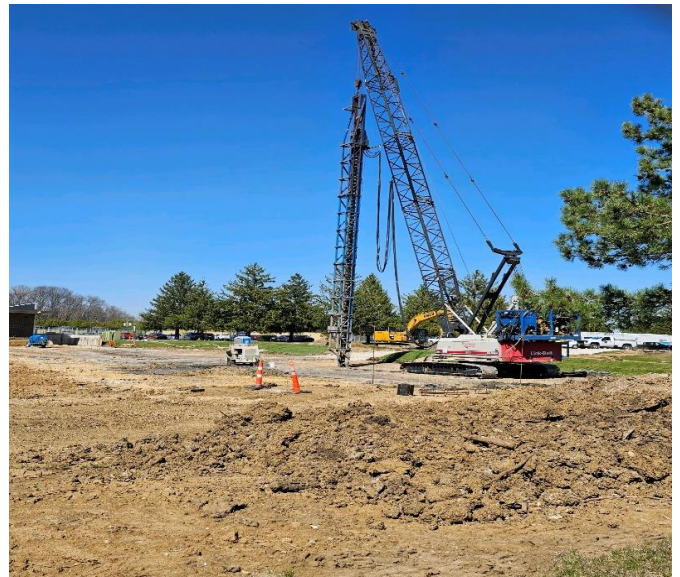
Piling tests on concrete for new building
