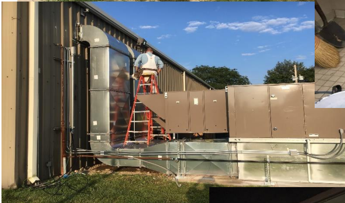
The Main Campus – PHS Building AA HVAC Replacement
