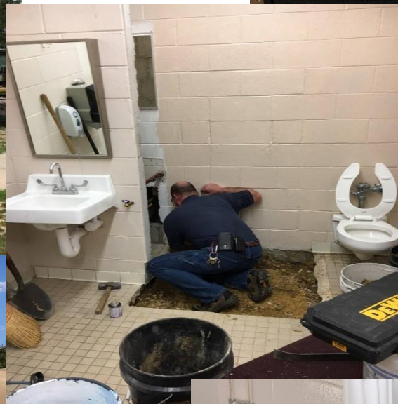
The Main Campus - Men's locker room shower area
