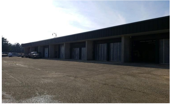
Bldg B Automotive east side of building
